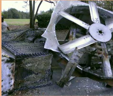
Virtually outside the conference room doors, workers dismantle the Crowne Plaza's old cooling tower while a new one was getting installed. Hard water had destroyed this 200-ton Marley. Industrial ScaleBlaster units are getting installed on the new cooling tower.
